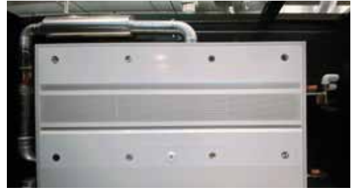
Figure 91: Ceiling-integrated chilled beam with air and chilled water supply
