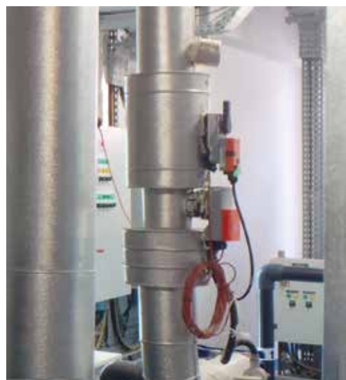
Figure 90: The supply of the fan coil units is equipped with the Belimo Energy Valve™
