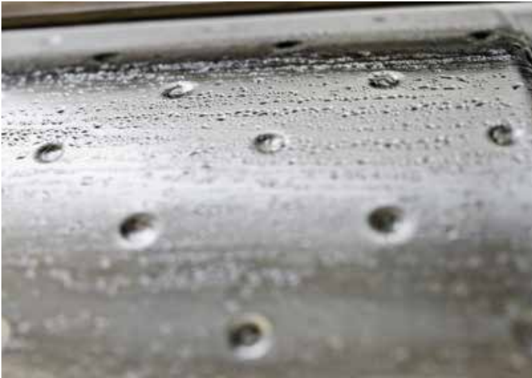
Figure 95: Condensation of humid air on the cold coil surface. The supplied cooling water needs to be above the indoor dew point to prevent condensation
